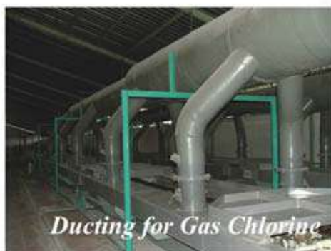
Pipe for Gas Chlorine
